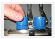
One circuit at a time, open the blue return valve to allow air to escape for 15 minutes. When finished, close the blue valve for the circuit and repeat Step 6 for the other circuits.
