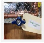
Connect a bleed hose or place a pail on the purge valve located under the pump. Put the liquid back in the injector.
