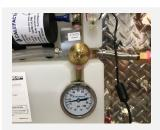
Once you are finished bleeding all circuits, make sure the injector brings the system pressure to between 12 psi and 15 psi. Refer to the dial on the injector. If the pump stops when the pressure on the injector control by turning it in the direction indicated.
