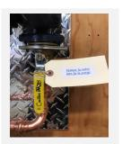
Close the ball valve at the pump inlet.
