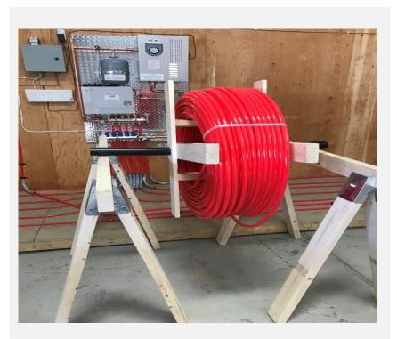
To change the tubing roll, simply unscrew the cross-shaped piece installed in step 10 and redo steps 10 through 14.
